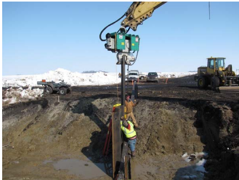
Photo Caption: Driving steel sheet-pile for a water control structure on Curtis Lake. Photo courtesy of Brad Karel, DU construction manager.
